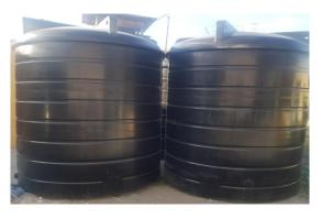
A bank of fifteen 2000-gallon tanks will be installed to provide storage for 30,000-gallons of purified water for distribution into the main water line on the campus.
